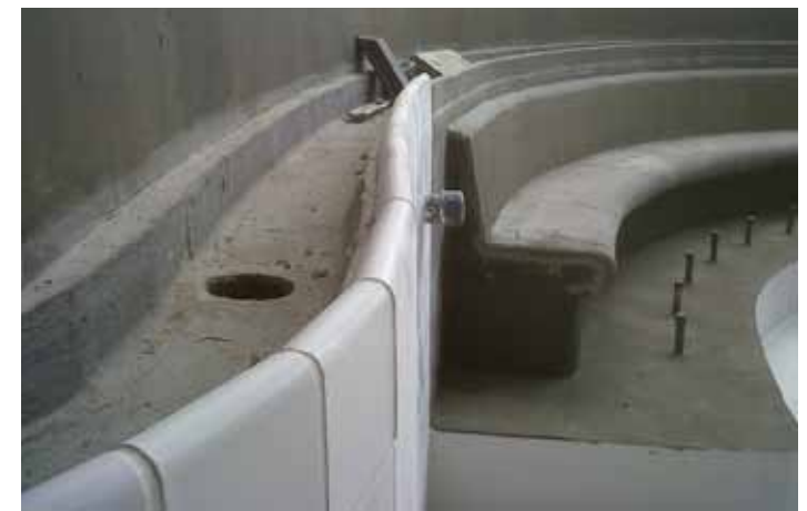
Sistema S9 Wiesbaden / Acquaworld / Concorezzo, Italy
